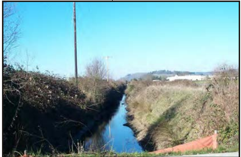
Muddy Creek Irrigation Channel
