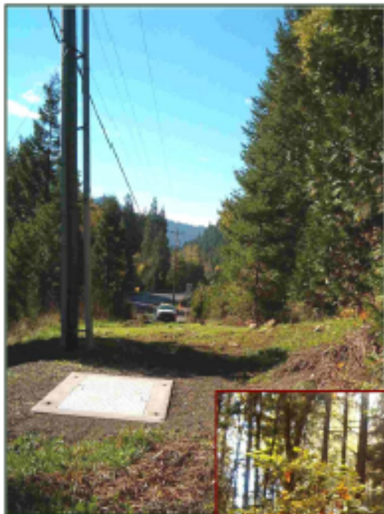
Top: Connection from overhead power to vault.
