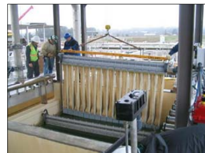
MEMBRANE TANK: CONTAINS THE POROUS FIBERS THAT SEPARATE THE TREATED CLEAN WATER FROM THE SEWAGE. THE MEMBRANES ARE FILTERS, WITH PUMPS DRAWING WATER THROUGH THE FIBERS LEAVING THE BUGS BEHIND
